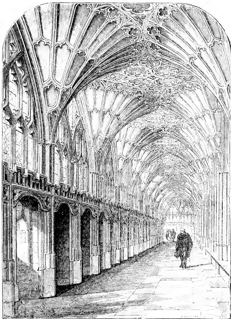
THE SOUTH ALLEY OF THE CLOISTER AT GLOUCESTER, SHEWING THE MONKS' CARRELS.
